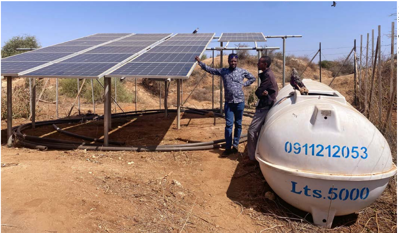
The solar panels powering the pump at Gadulicha ela (deep well) in Dhas kebele .
